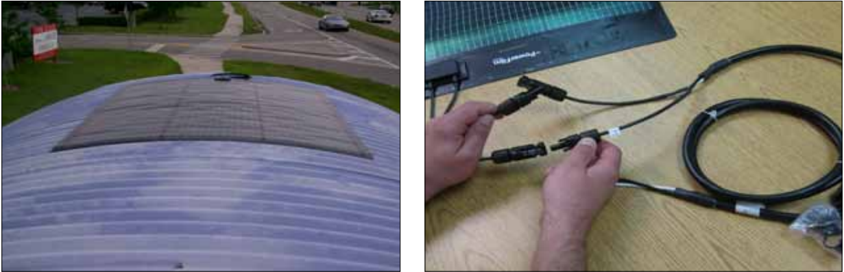
FIGURE 14 CONNECTING MC CONNECTORS
