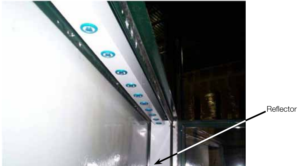
FIGURE 19 INSTALLING LED LIGHTBAR
